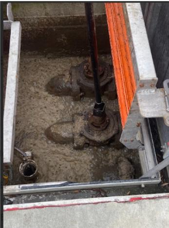
The 6" plug valve for wasting in train 2 (pre-anoxic) was inoperable. Tomar is scheduled to be onsite on November 1st to make the necessary repairs. Tomar repaired the wasting valve.
